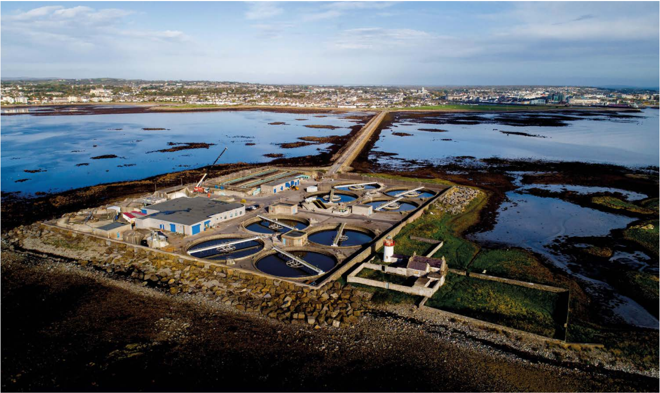
Mutton Island wastewater treatment plant, Galway Bay Courtesy of Irish Water/Uisce Éireann
